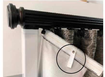
Notice the Ripplefold clip on the drapery panel. Do not do this. Be sure the clip is attached to the drapery track before attaching the fascia.
