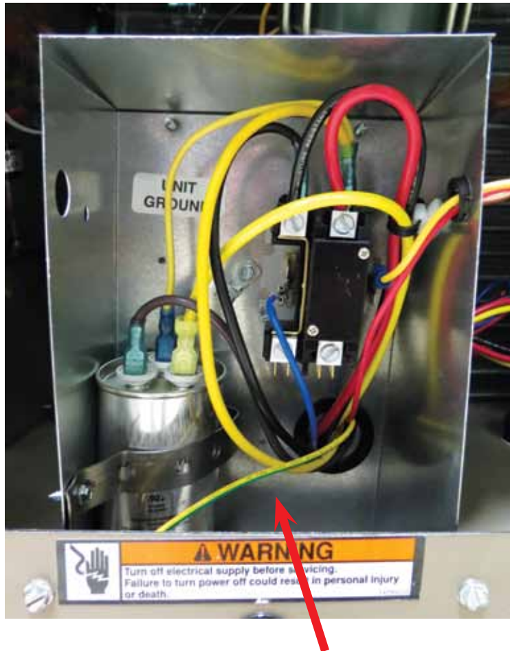
Condensing Unit Control Box
