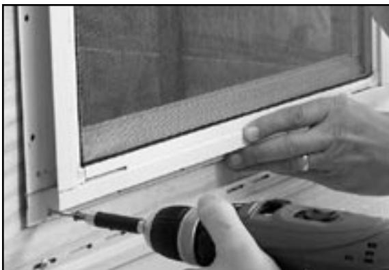
Keeping the window level, install a #8 x 1/2" screw into each of the predrilled holes of the window flange (32 places).
