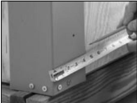
**2****Place a corner post against the frame corner, allowing the bottom to rest on the rim joist. Align the edge with the measured and marked lines from step #1. Install a screw at the nailing strip as shown:**
