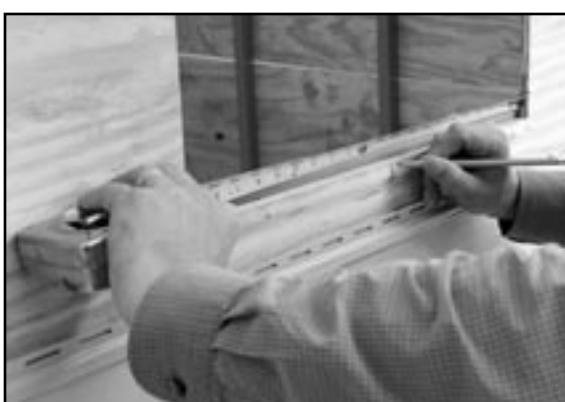
Place the window into the opening (screen to the outside). Align the center hole in the bottom flange of the window with the marked center of the cutout and level the window.
