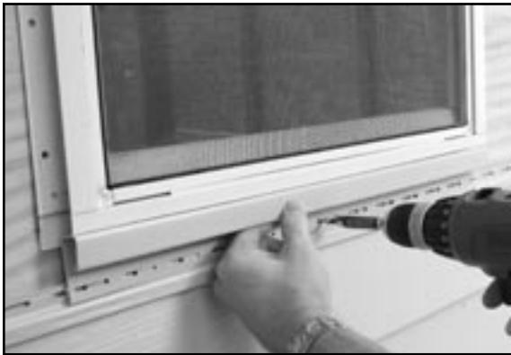
**NOTE:** The J-channel must be installed around the window before any more siding is attached.
