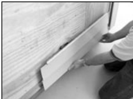
**NOTE:** There should be about 1/2" gap between the end of the siding piece and the inside wall of the corner post pocket.
