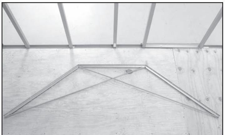
d. Use one #10-24 x 1-3/16" Oval Head Bolt and #10-24 Nyloc Nut to assemble Diagonal Braces.
