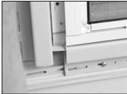
This screw should be installed at the top of the slot to ensure the J-channel does not slip downward
