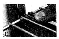
After all shelves are positioned properly, lock Shelves into Brackets by sliding the plastic locking clip towards the back wall. It will "SNAP" into locked position.
