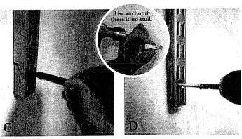
Mark bottom hole of each Upright. Drill 1/8" pilot hole into stud. (Use Wall Anchor and 3/8" bit if there is no stud.)
