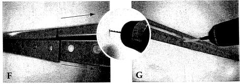
Slide second Hang Rail to the right wall of the closet, and then back it away from the right wall until the holes in the two Rails line up. Repeat Step C to secure to the wall.
