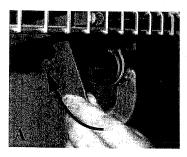
Install Rod Hanger into bottom of Bracket by tilting it backward until it locks in place.
