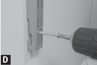
Fasten screws Drill 1/8" pilot hole and fasten both screws (use wall anchor and 3/8" bit if there is not stud). To position the second upright extension, use 22" rail cover to ensure proper spacing is parallel from the first upright extension.
