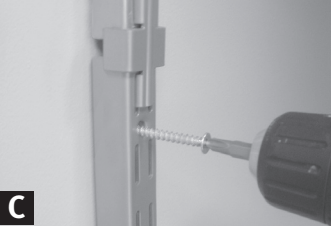
Fasten screws Drill 1/8" pilot hole and fasten both screws (use wall anchor and 3/8" bit if there is not stud). To position the second upright extension, use 22" rail cover to ensure proper spacing is parallel from the first upright extension.
