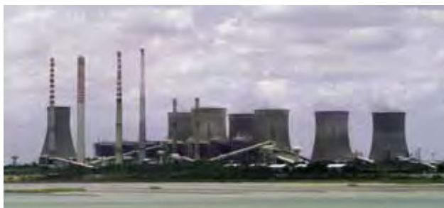
Raichur Thermal Power Station - Raichur, India
