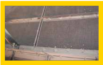
Conforma Clad screens after nine months.
