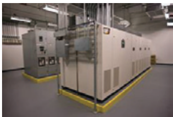
Flywheel UPS & Paralleling Switchgear
