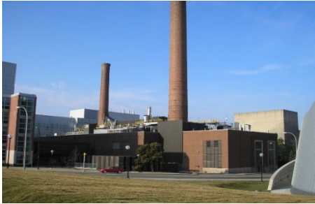
Central Power Plant, Univ. of Michigan
