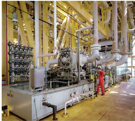
**Figure 8-9.** Flash gas compression and reinjection.
