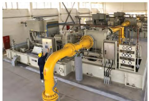
**Figure 7-6.** Electric-motor drive package: VFD controlled motor driving the compressor via a speed-increasing gearbox.
