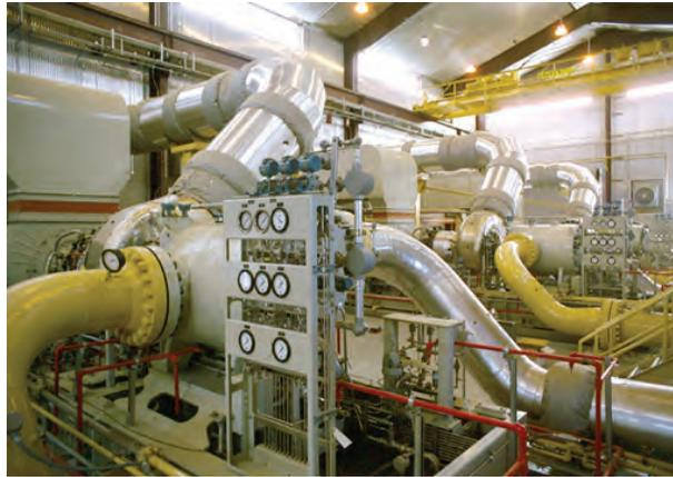
**Figure 8-21.** Pipeline compressor station with three compressor trains in parallel.
