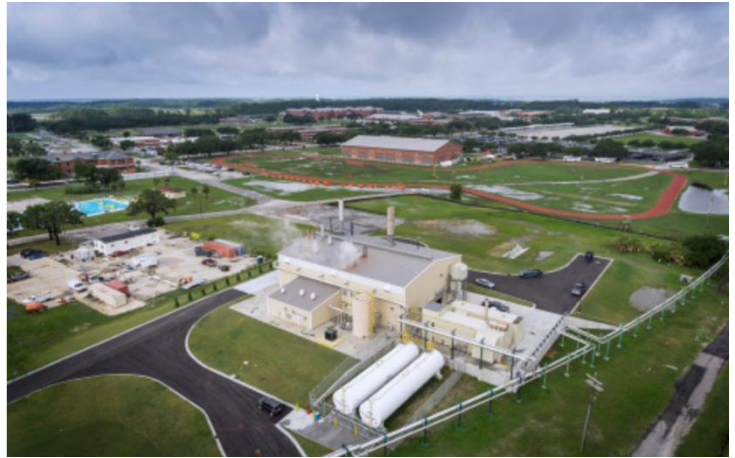
MCRD's new central plant with microgrid and island mode capability providing 3.5 MW of electric and the full steam load required by MCRD Parris Island. Photo courtesy of Business Wire
