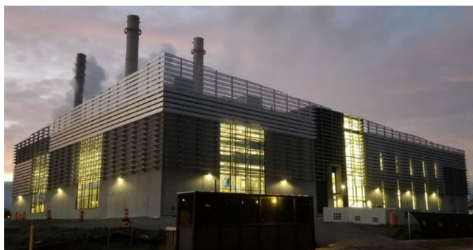
Ford REC's New Energy Plant: Source DTE Energy Services
