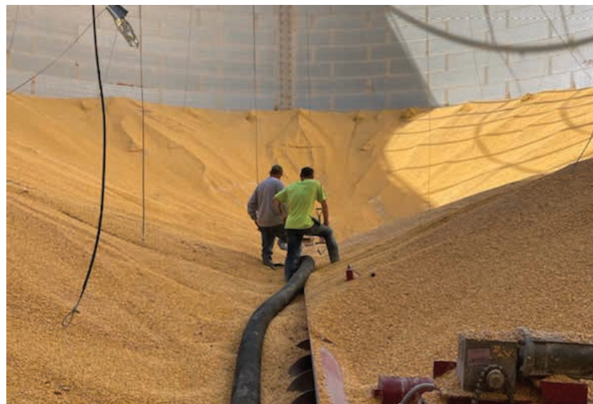
Salvage operation at Mayfield Grain.
