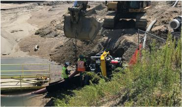
And in the spirit of making operators' days more simplified, Atlas Copco also lowered its pump profile with the PAS 200 / PAC F88, which are powered by the Perkins® 904J-E36TA engine. Bringing the machine height down makes it significantly easier for users to physically manage the pipes and connections. The low profile even increases the performance of the pumps, since they gained an extra bit of suction lift by being closer to the ground.
