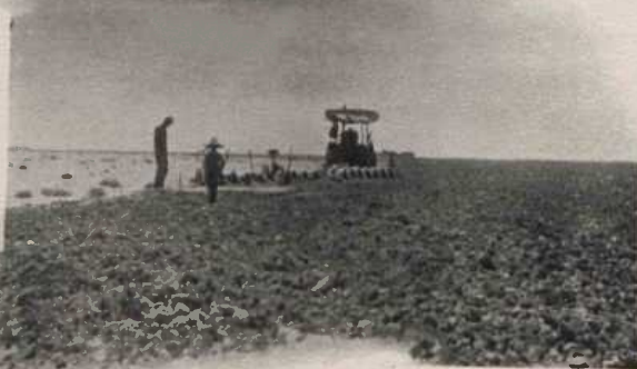
Pulling 14 feet of Plows with Harrows
