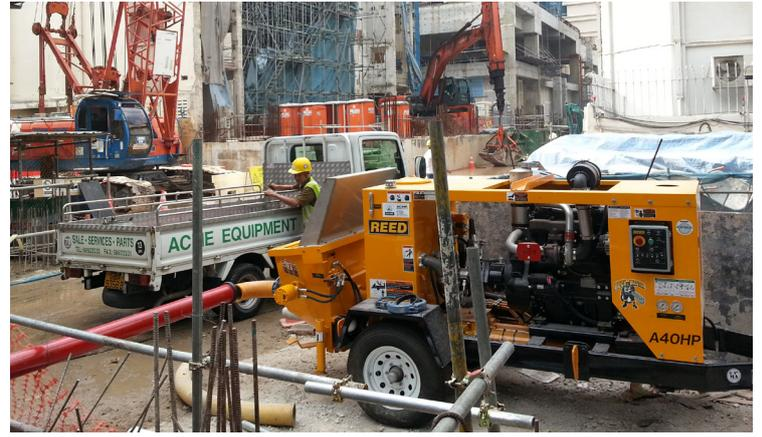
The A40HP features a variable displacement hydraulic pump that includes an extra flow-control valve, allowing users to adjust the output while keeping the engine's RPMs constant. And this one's got serious power. It's rated at 40 cubic yards per hour, while offering up 1172 psi, 82 bar when it comes to concrete pressure—which means it can pump higher, further and faster than the others in the series.
