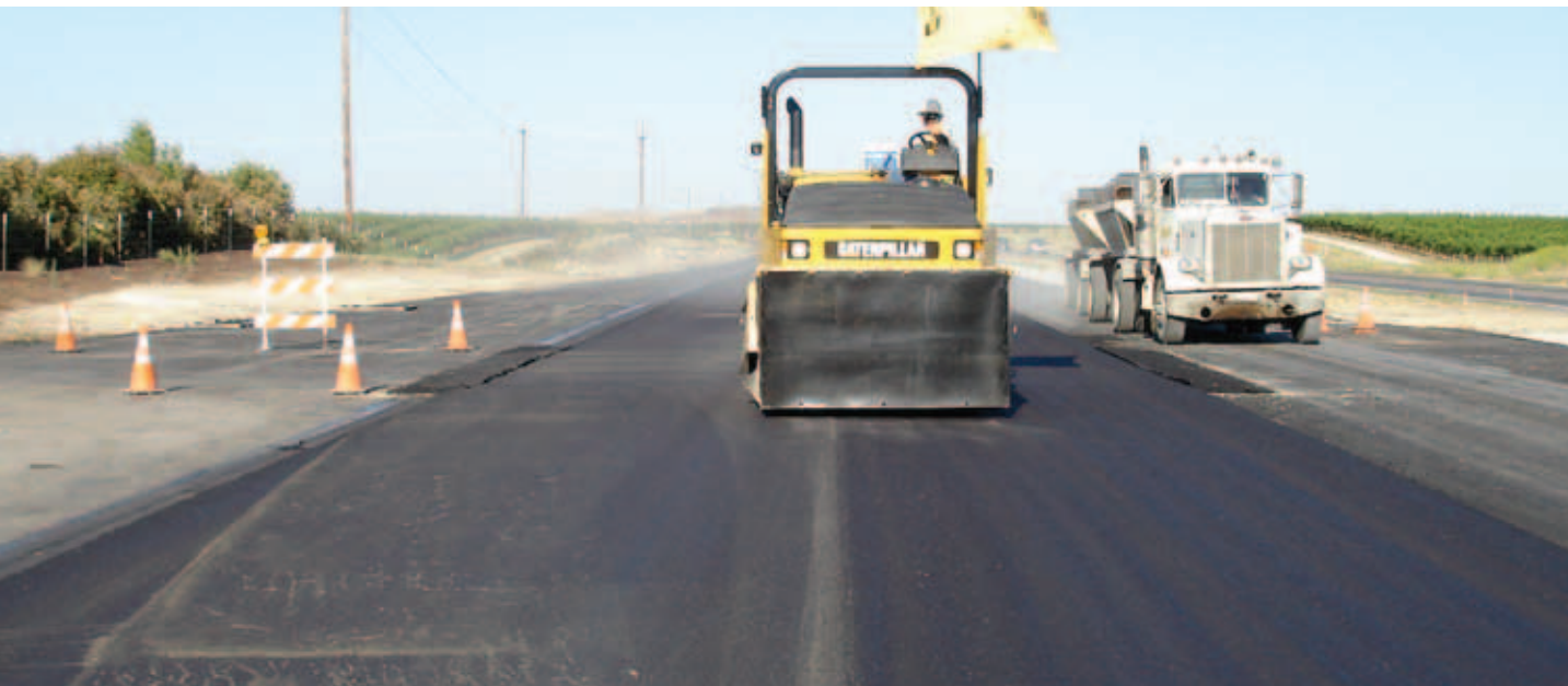
Pneumatic compactor sealing a hot / cold longitudinal joint.
