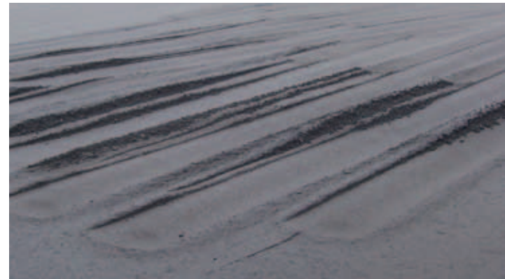
Deep tire marks created by operating on a thick layer composed of a tender mix will be difficult to clean up.
