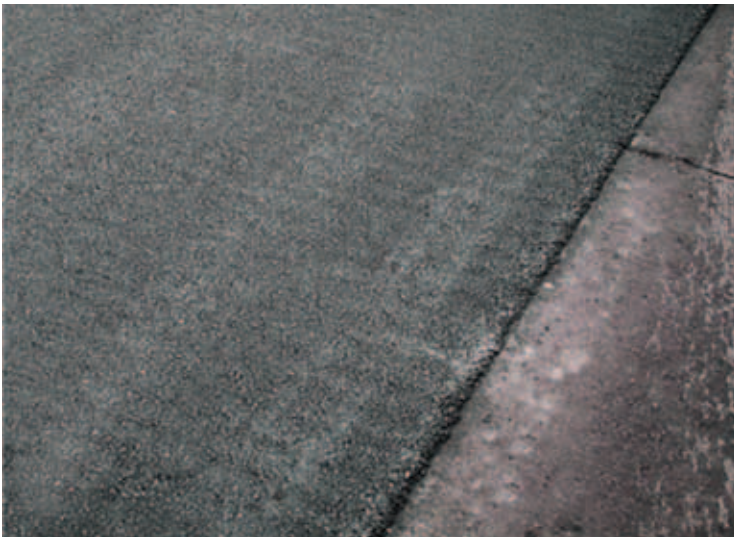
Drum impact marks, above. At right, establish a pattern that does not distort the hot asphalt when reversing.
