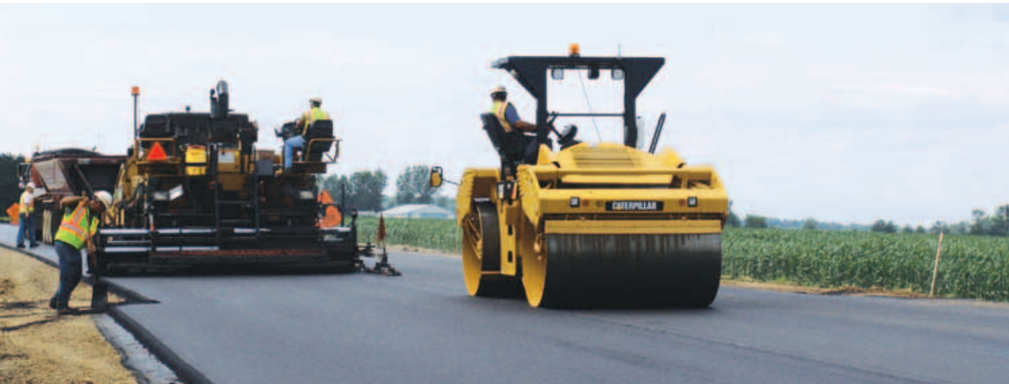
Sealing the longitudinal joint during the first pass improves the appearance of the joint.
