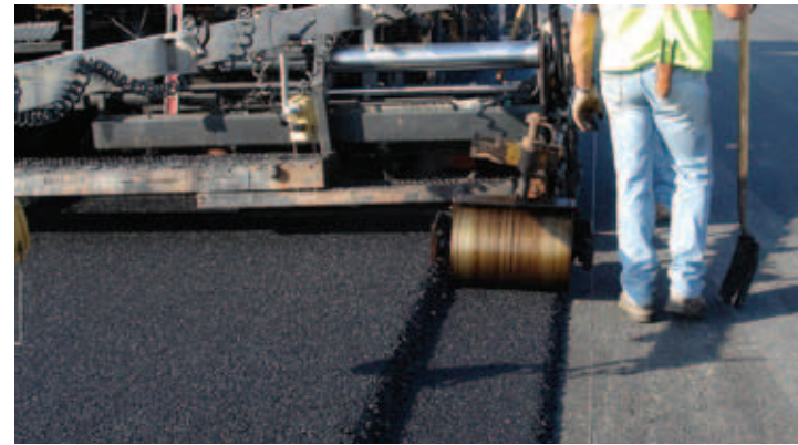
Towed rollers may be used in conjunction with notched wedge joints.
