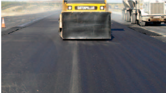
Pneumatic compactors in the intermediate phase are effective at sealing hot / cold longitudinal joints.
