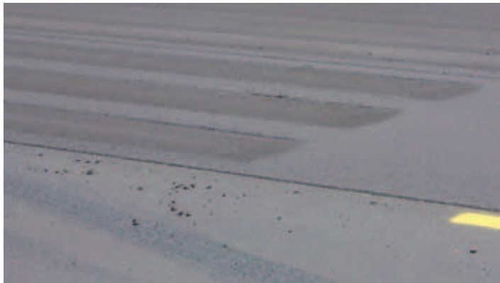
Tire marks left by the pneumatic compactor can normally be cleaned up by the finish-phase compactor.
