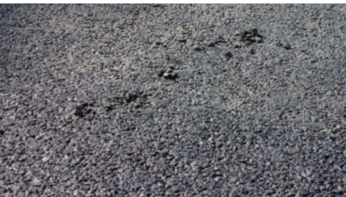
Divot made in the fresh mat by asphalt stuck to the drum.
