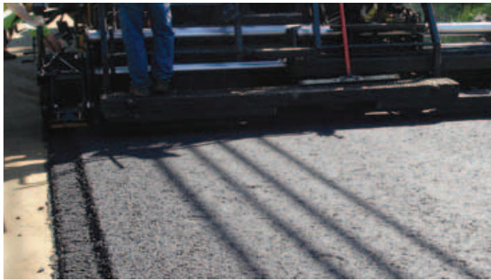
A notched wedge joint being laid down by the paver.
