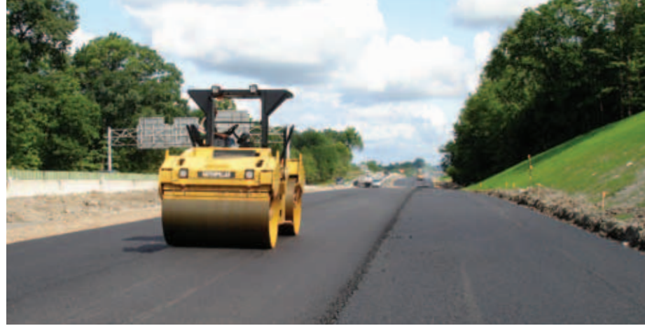
Tandem drum rollers operated in the static mode are common during the finish compaction phase.
