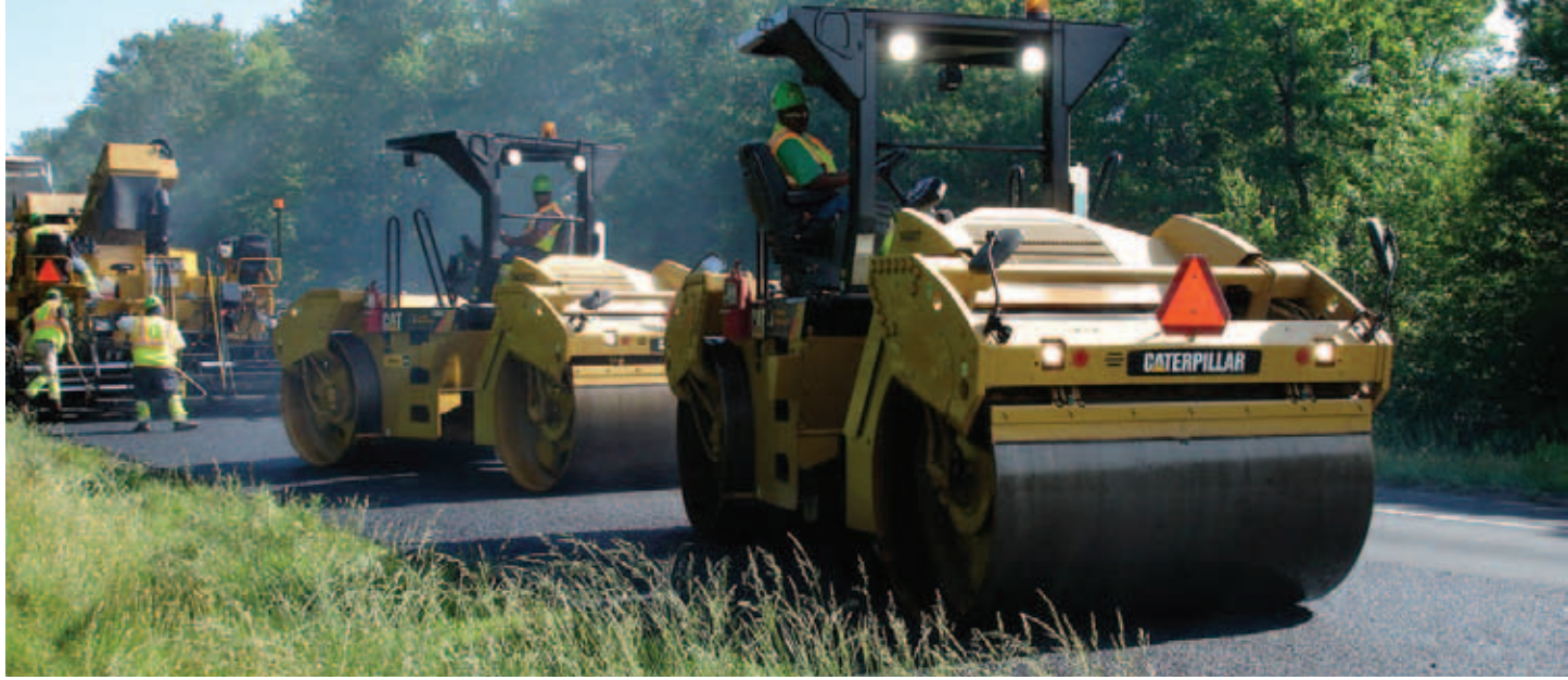
Two initial phase compactors reversing direction behind a paver. Note angled stop.
