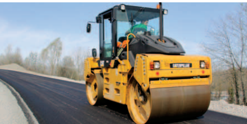
Steel drum, vibratory rollers are commonly used for initial compaction.
