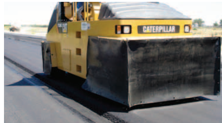
Pneumatic compactors always stay at least 15 cm (6") from unconfined edges.
