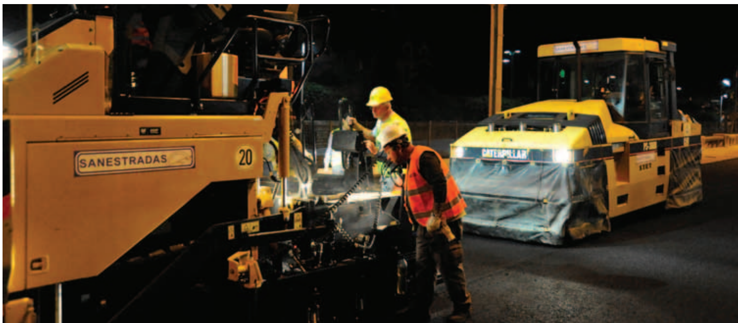
Pneumatic compactors can exert high forces without delivering impact forces.
