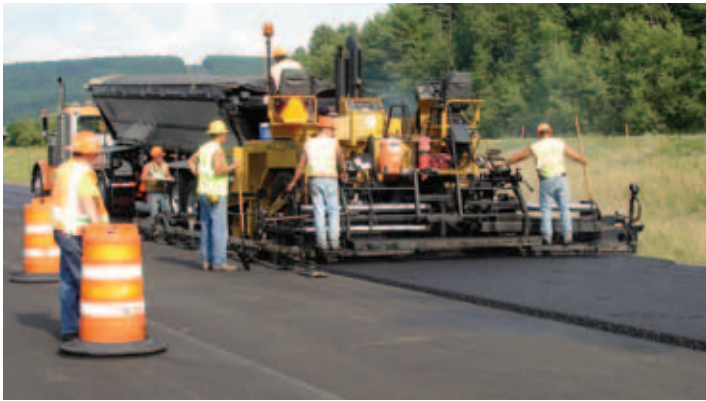
Create a vertical unconfined edge by running the screed end gate in the float position on the grade being paved.
