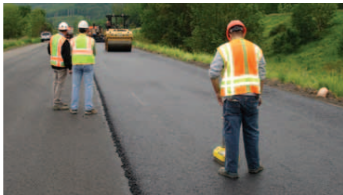
Asphalt compaction is started by the paver screed and finished by compactors working immediately behind the paver. Crew members often monitor the compaction process.
