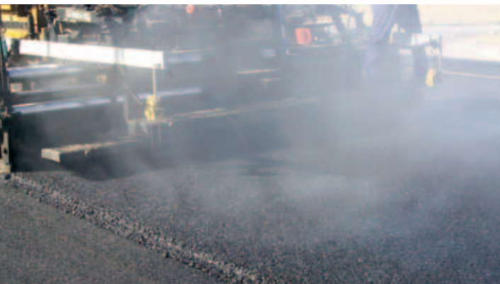
Asphalt compaction is started by the paver screed and finished by compactors working immediately behind the paver. Crew members often monitor the compaction process.
