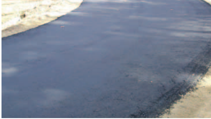
Conventional 170 cm (67") drum compactor rolled continuously around the radius.
