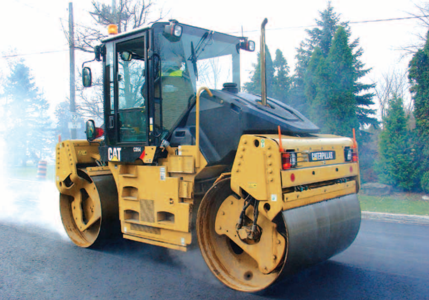
Cat CD54 working in the initial phase of compaction.
