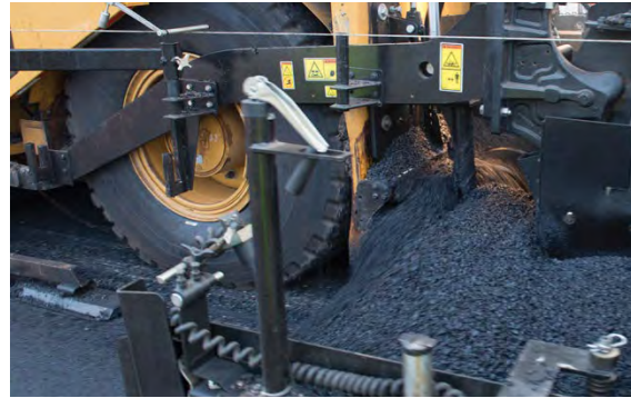
Mechanical or sonic sensors have equal accuracy using the ski stringline as a guide.
