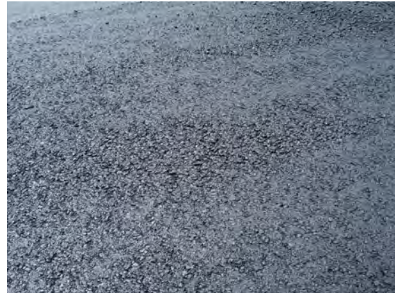
Random patch segregation caused by running the mix level low in hopper insert.
