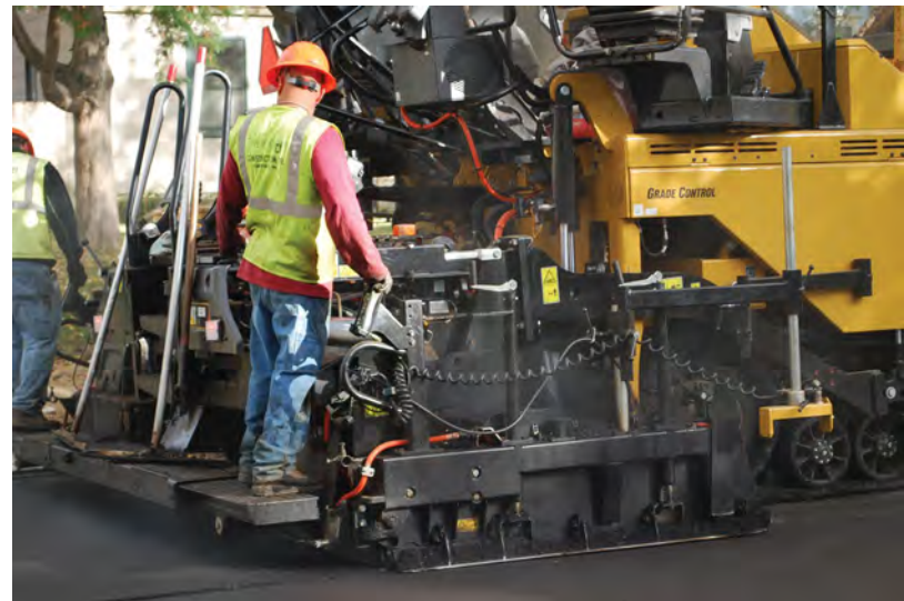
A single grade sensor installed close to the auger chamber provides the best control of layer thickness and yield.
