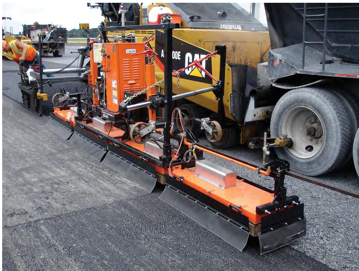
Pre-heating the cold, compacted layer is specified on some applications.
