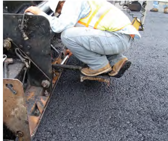
The angle of attack on screed extensions should be adjusted while the paver is moving.
