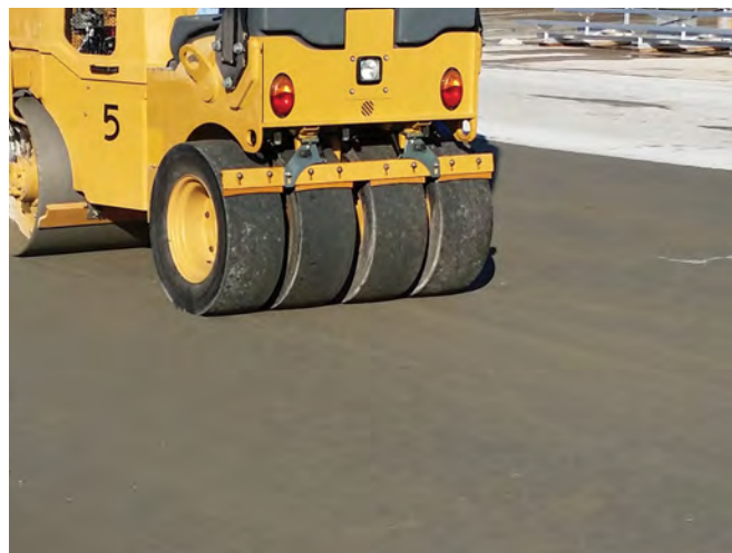
Straddle the longitudinal joint when making the first pass forward.
