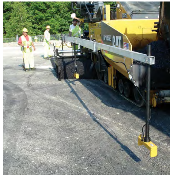
Cat non-contact ski setup to reference grade inside the paving width.
