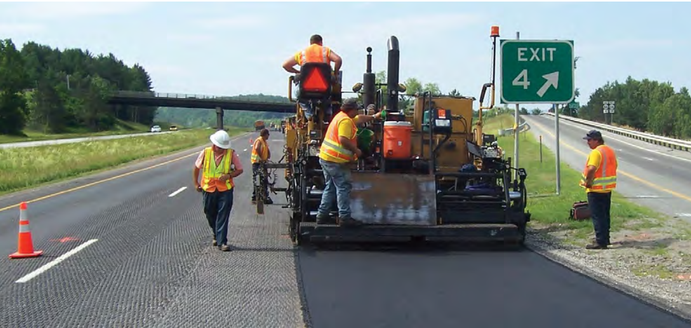
Paving emergency lanes first improves the smoothness of adjacent driving lanes.
