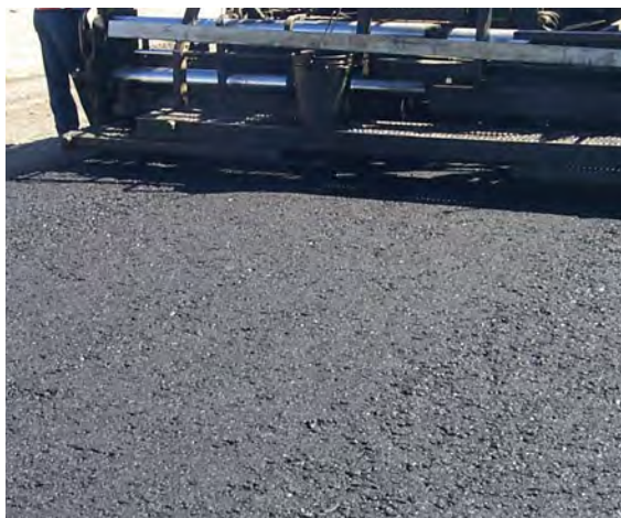
Random patch segregation can be seen and also detected in thermal images.
