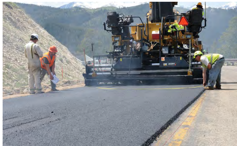
Left and right hydraulically extendable screed extenders simplify the task of changing paving width.
