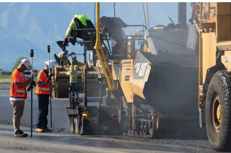
On airport projects, elevations and yield are often the most critical requirements.
