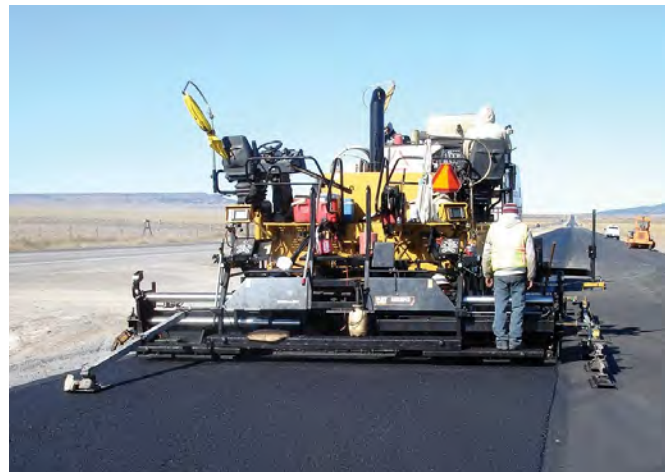
Dual, mechanical averaging skis can produce up to a 60-70 percent improvement in one-pass smoothness.
