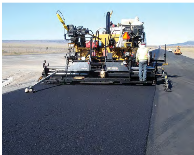
Joint matching with averaging skis is common when there is a ride quality specification and the adjacent layer is reasonably smooth.
