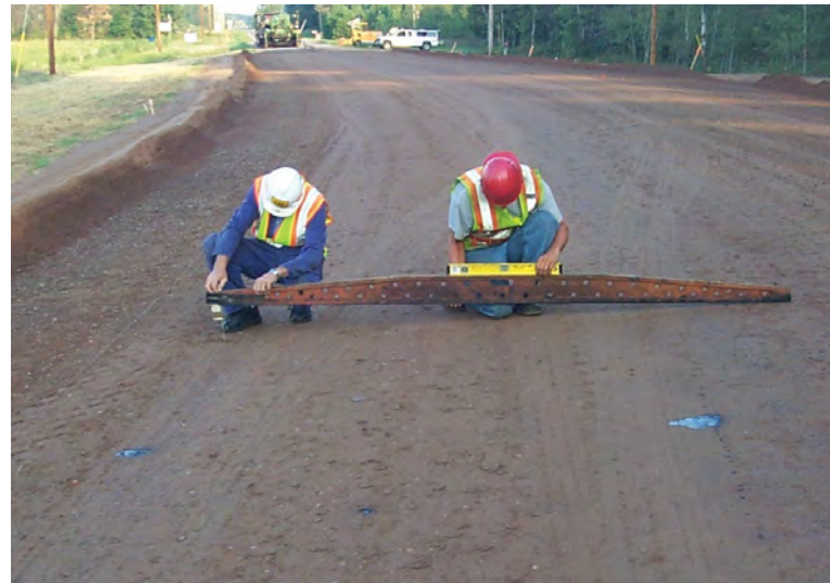
Check slopes throughout the length of the superelevated curve.
