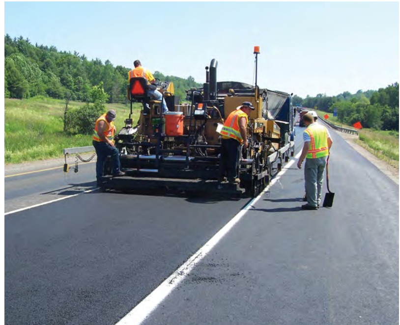
Averaging ski using emergency lane as a grade reference.
