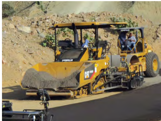
Roller-compacted concrete can be transferred to the paver by an end dump truck or by a cement mixer truck.
