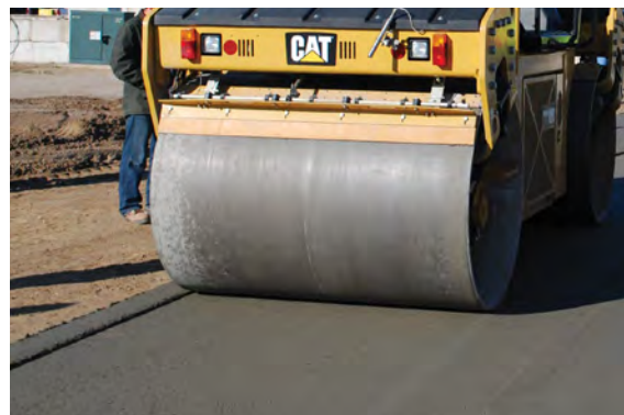
To avoid deforming the edge, stay away from the edge 30 cm to 40 cm (12" to 15").
