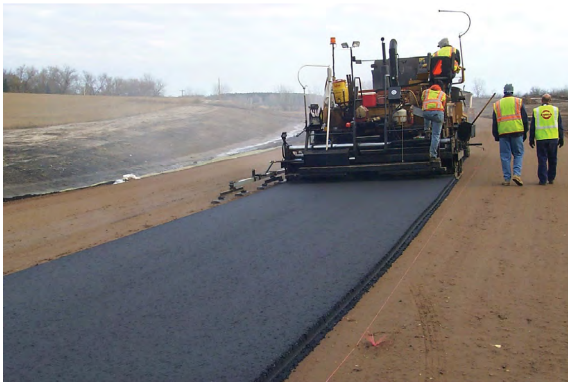
Paving superelevation with averaging ski on left, slope right.
