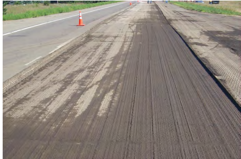
Paving over a high spot in the grade will create texture differences in the surface of the asphalt layer.
