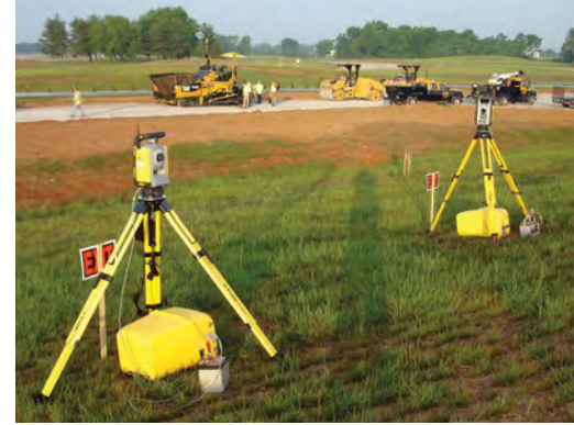
Machine targets on the paver are tracked by the Universal Total Stations.
