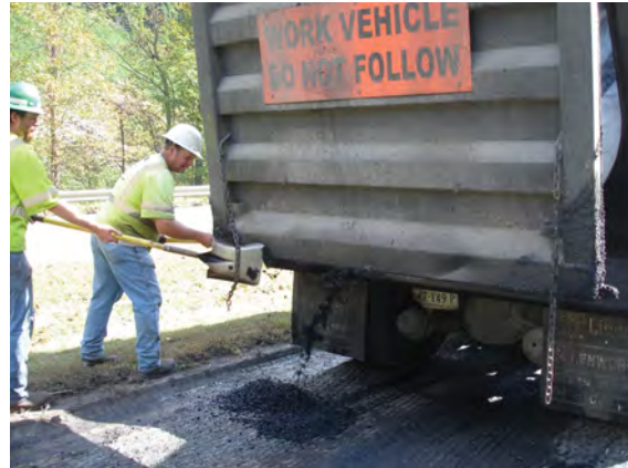
Truck clean-out should not occur in front of the paver.
