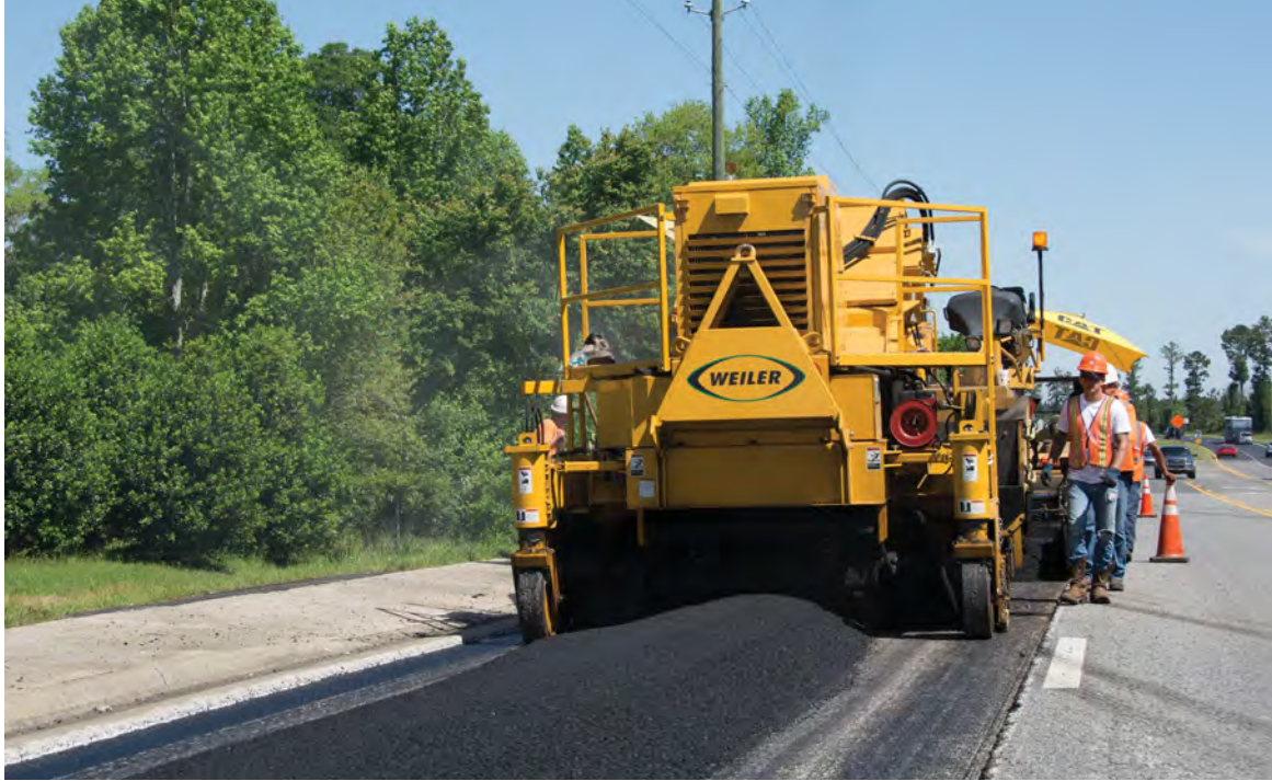
High-production windrow elevator transferring material into a paver with hopper insert.
