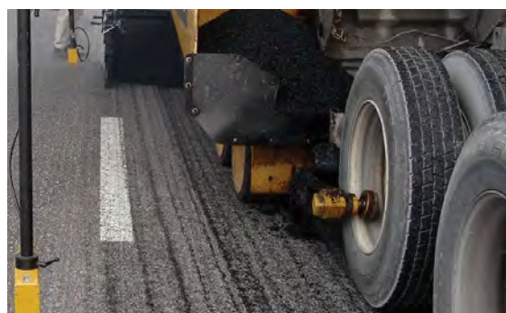
A truck hitch provides a positive connection between the haul unit and the paver.
