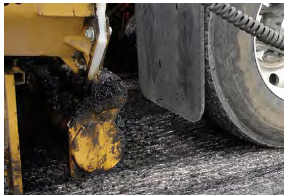
The truck always stops short of the push rollers.
