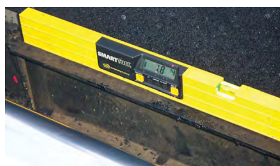
Verify the actual slope of the screed.
