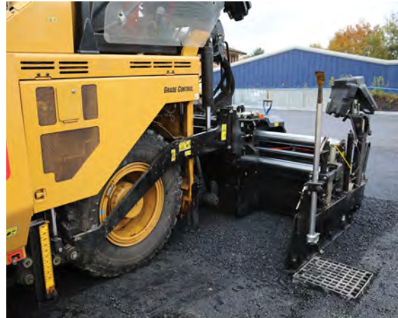
Drainage and appearance are important to the owners of parking lots.
