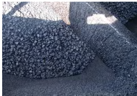
Segregation can occur in the hopper insert.
