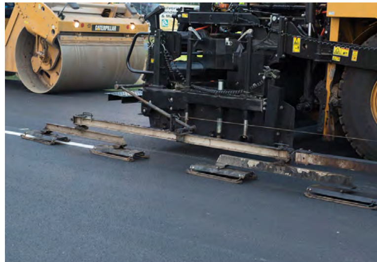
Mechanical averaging skis are often used to help meet ride quality specifications.
