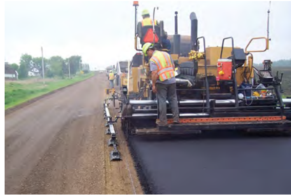
9-meter (30') multi-articulated, outboard leveler used to improve an extremely rough grade.
