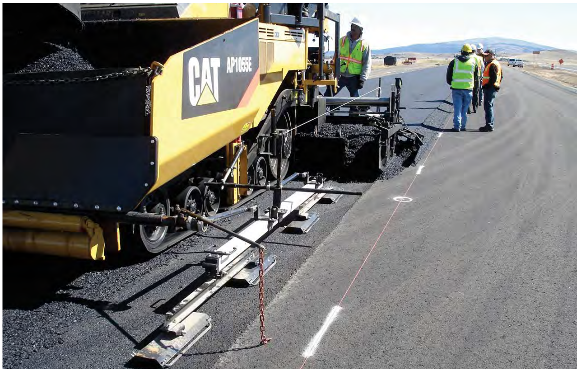
Cat 9-meter (30') Fore 'N Aft Leveler provides averaging capability inside the paving width.
