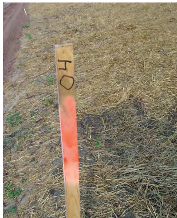
Grade stake showing slope at a point in the superelevation runoff.
