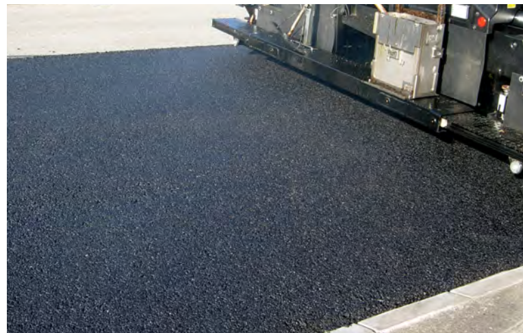
The texture of the mat is influenced by the type and size of the aggregate.
