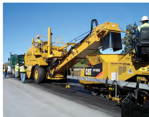
Material blending by the material transfer vehicle improves control of segregation, uniformity and layer temperature.
