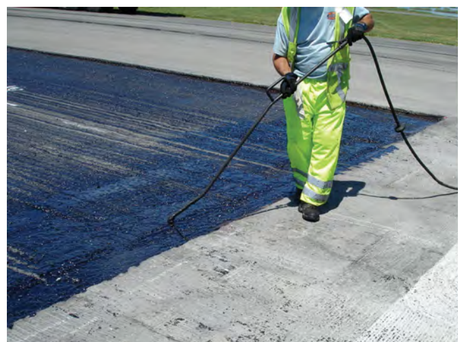
Use a spray wand or hand applicator to apply tack to the face of the butt joint.
