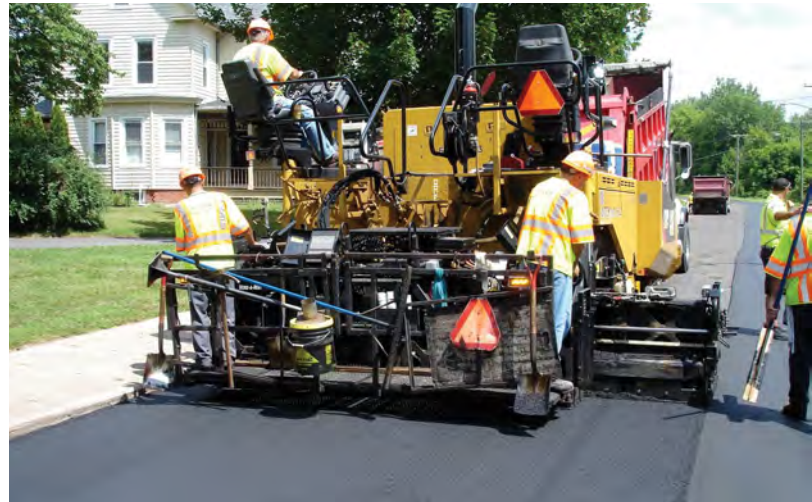
Screed plates of different lengths can cause minor texture differences.
