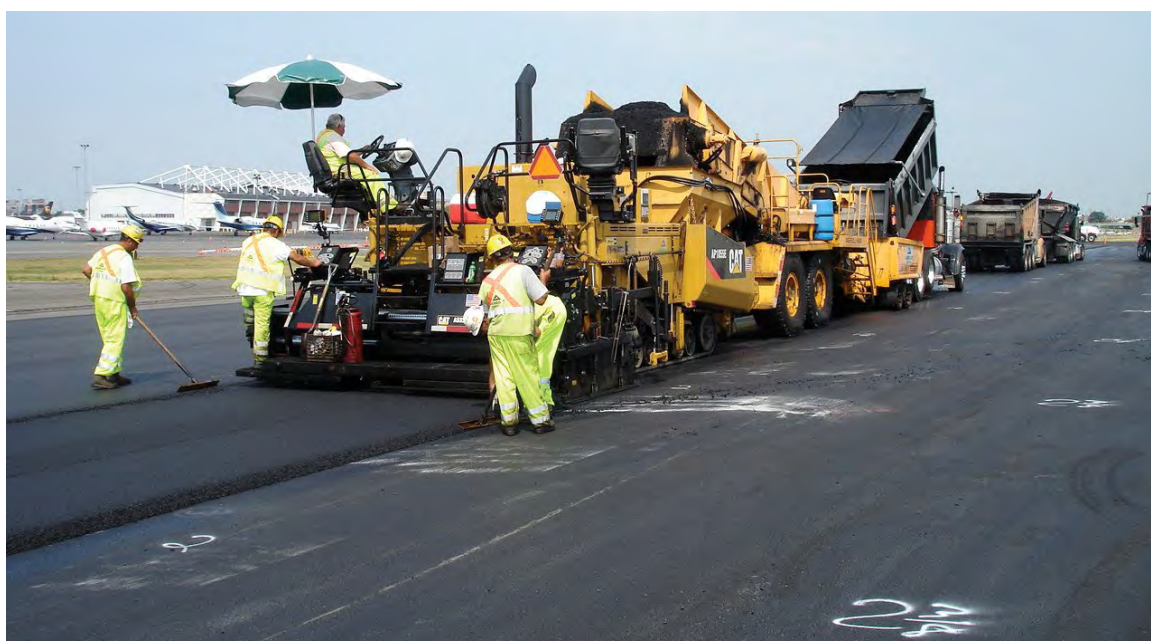
A survey crew may mark elevations directly on the grade in a grid pattern.
