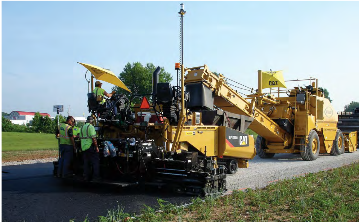
Cat Paver equipped with Trimble three-dimensional guidance system.
