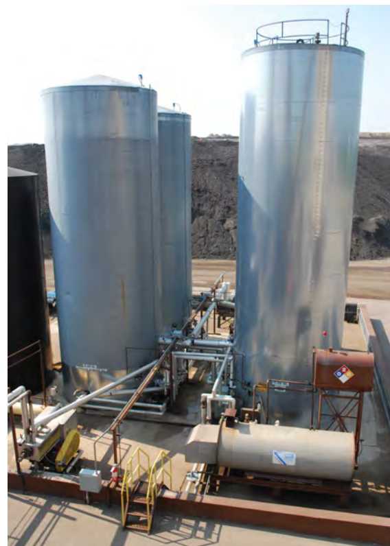
Heated bitumens added to the mix provide the required binder.
