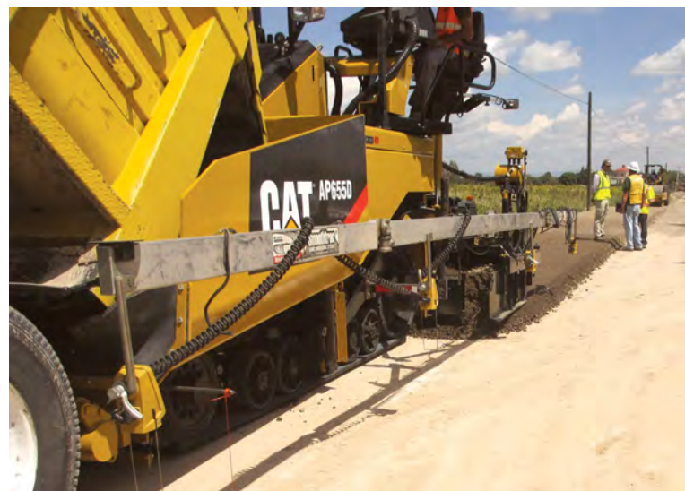
Conventional grade and slope control provides precise depth and transverse profile.
