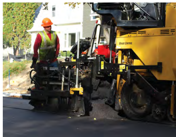
A single sensor is often used for height match on a longitudinal joint in parking lots and streets.
