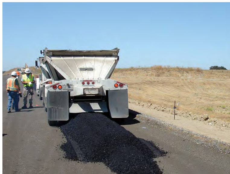
Various types of haul units can be used to create windrows.
