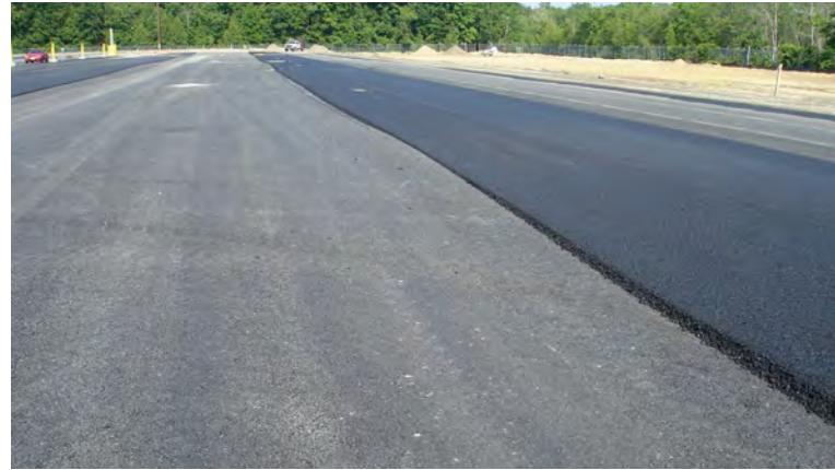
When averaging skis are used, the screed tends to fill in low spots and level off high spots with yields varying accordingly.
