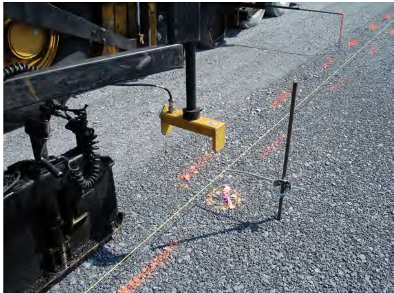
Cat Grade Sensor in stringline orientation.
