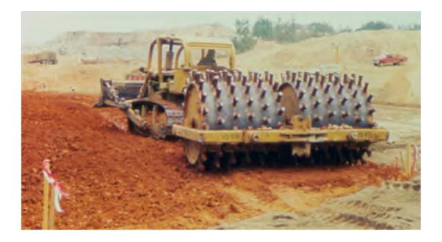
The pads on sheepsfoot drums penetrate through the top lift and actually compact the lift below. When a pad comes out of the soil, it kicks up or fluffs the material. The result is a loose layer of material on top. When more fill is spread, the top lift will be fluffed and the previous layer will be compacted. A sheepsfoot compactor truly compacts from the bottom up.
