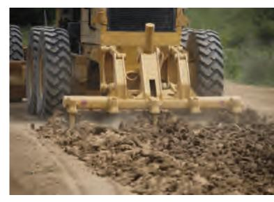
When moisture content is too high, opening up the soil speeds drying time.
