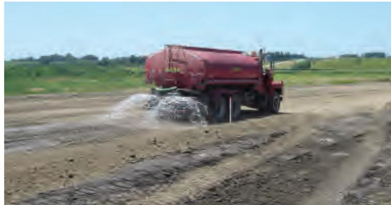
the load-bearing capability of the structure. The particles will also be over-lubricated, allowing them to easily displace.
