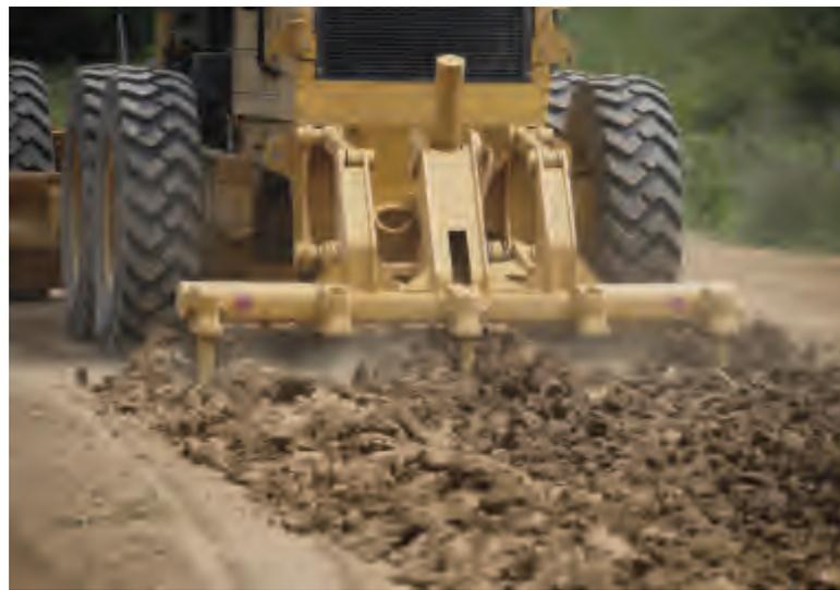
*When moisture content is too high, opening up the soil speeds drying time.*
