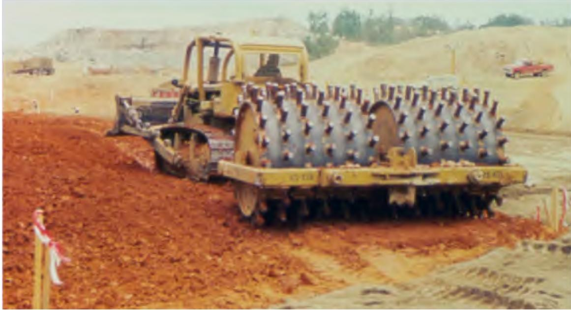
The pads on sheepfoot drums penetrate through the top lift and actually compact the lift below. When a pad comes out of the soil, it kicks up or fluffs the material. The result is a loose layer of material on top. When more fill is spread, the top lift will be fluffed and the previous layer will be compacted. A sheepfoot compactor truly compacts from the bottom up.
