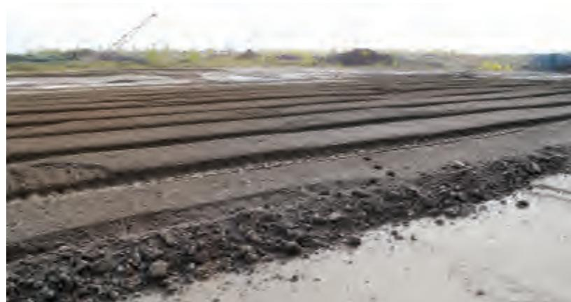
**Compactive Effort** – Compactive effort is the amount of energy imparted to the soil in order to rearrange and compact the soil particles. Varying machine parameters such as weight, width, tire pressure, vibration amplitude and frequency can change compactive effort. Some of these parameters can be adjusted on a single machine. Others, such as width, may require a different machine in order to alter compactive effort. Certain magnitudes of these parameters are necessary for any given project.
