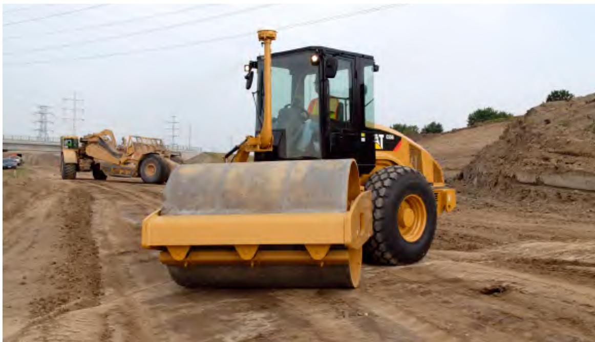
*Proofing Mode* – Once production compaction has been completed, the compaction measurement system can be used as a proof compactor to verify the quality of the work in this more precise mode of operation. This approach is intended for use when the contracting authority is requesting documentation or a map showing an accurate indication of ground stiffness for a particular phase of construction.
