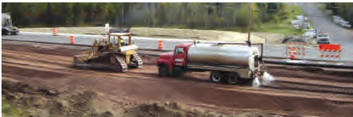
*When moisture content is below the optimum, water may be added to ensure that proper compaction can be reached.*
