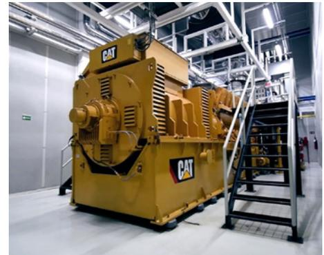
*The cogeneration plant has two Cat® CG260-16 gensets that produce a total of 8 MW of electric power and one absorption chiller, which produces 988 tons of chilled water for air conditioning.*
