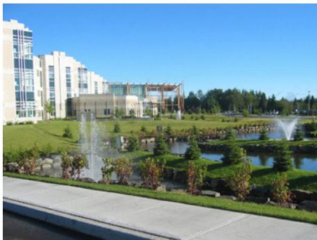
With a daily average of 420 patients and 2,500 staff, the demand for electricity and hot water is constant at Thunder Bay Regional Health Sciences Centre in Ontario, Canada.
