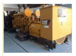
Generator sets ranging from 200 to 2,500 kVA have been installed to provide power for intelligent traffic systems and toll collections systems as well as providing power and lighting at road junctions, tunnels and services.
