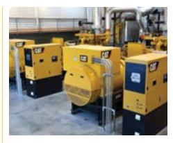
Located behind the new 17,000 square-foot office of Lehi City Power, the Broadbent Generation Facility first opened in March 2018. It has three Cat G3520H generator sets that produce 7.2 MW of power during times of peak demand, when energy prices are high.
