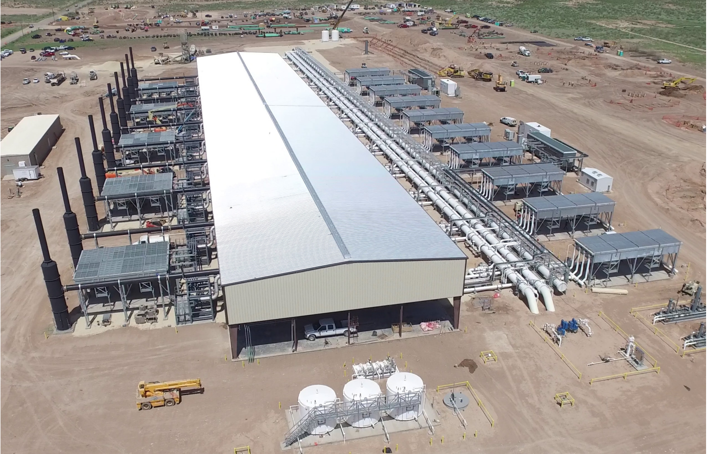
Waha Compressor Station - Energy Transfer Powered by G3616 A4 engines
