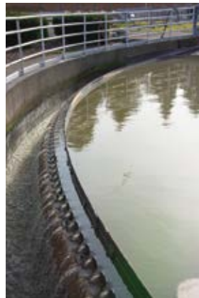
FOG collection tanks
