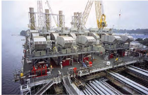
**Figure 5-4.** Gas Turbine Installation on an FPSO
