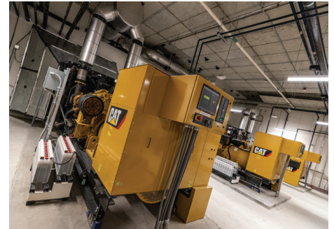
Cat® C32 diesel generator sets featuring high power density reduce total costs for site preparation, transportation and installation, while requiring less overall space.
