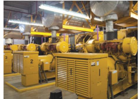
*Four Cat® 3512 diesel generator sets serve as emergency backup power for the life-safety systems and other operations of three hospitals and smaller facilities, ensuring a continuous supply of power.*
