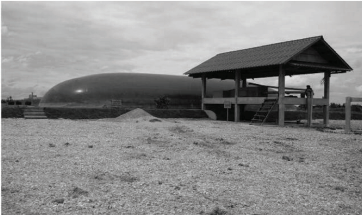
Figure 16: Buffer Tank and Digestion Process (Front) at Kampangetch Swine Farm, Thailand
