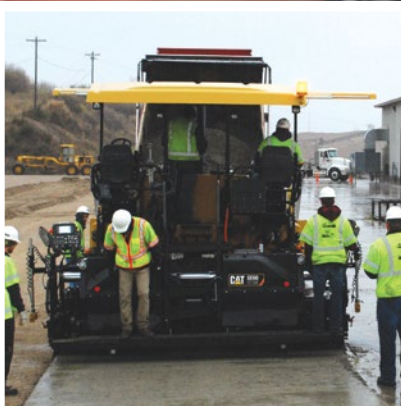
^ AP1055F/SE60 VT XW Mistura de RCC (Roller Compacted Concrete, Concreto Compactado a Rolo)
