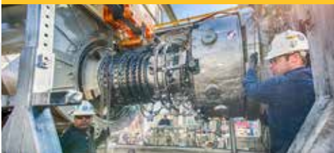
Turbine exchange performed on-site
