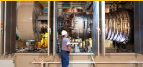
Parts prepared for next Solar overhaul
