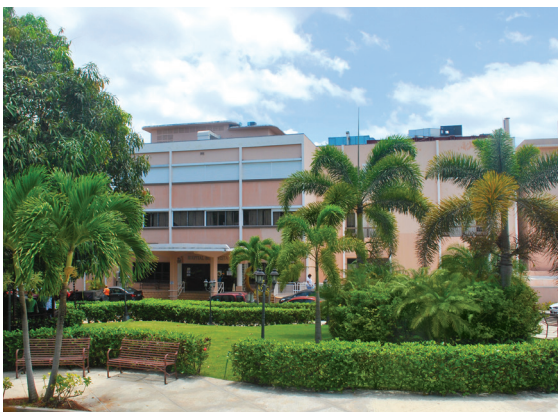
BELLA VISTA HOSPITAL – MAYAGÜEZ, PUERTO RICO
