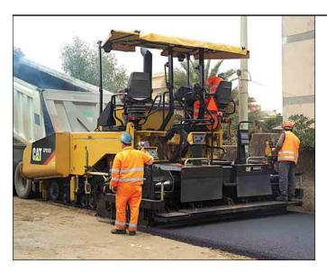
The AS4251C screed paves from 2550 mm to 5000 mm. With mechanical extensions added to both sides, maximum paving width is 8000 mm.
