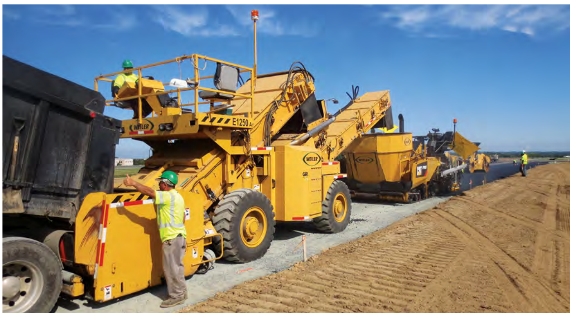
Efficient paving means continuous paving on highway projects.
