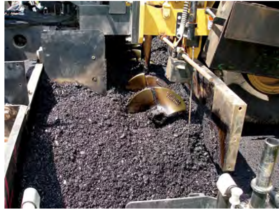
A well-trained crew has set up the feeder system to maintain the correct head of material.
