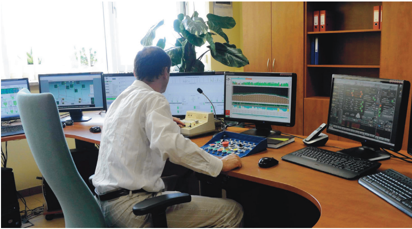
Surface control room.
