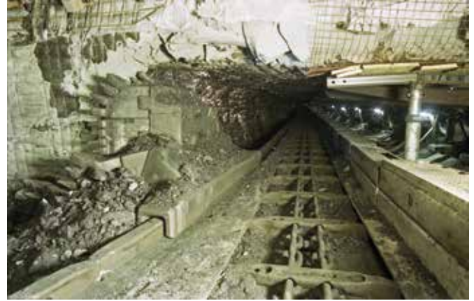
Plow at face end (tail drive)
