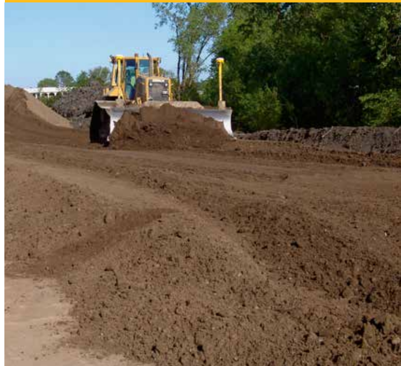
Constructing a test section.
