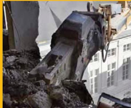
**Concrete Cutter (CC) Jaw**
