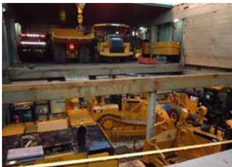
A narrow window of warm weather during the summer enabled machinery to reach the project site.
