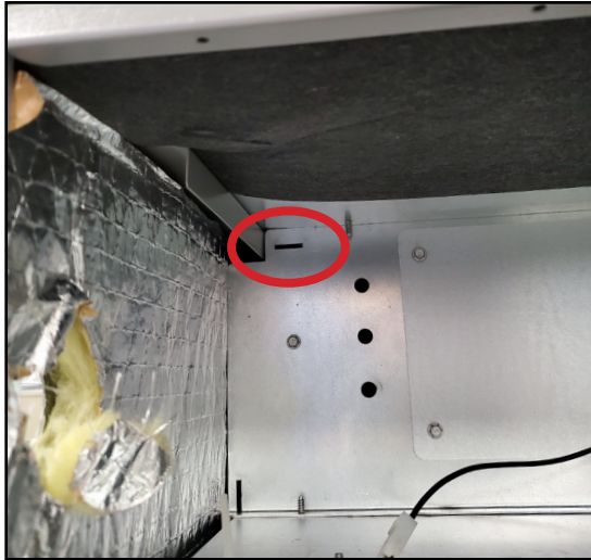
Figure 12. Notch for Control Panel Relocation
