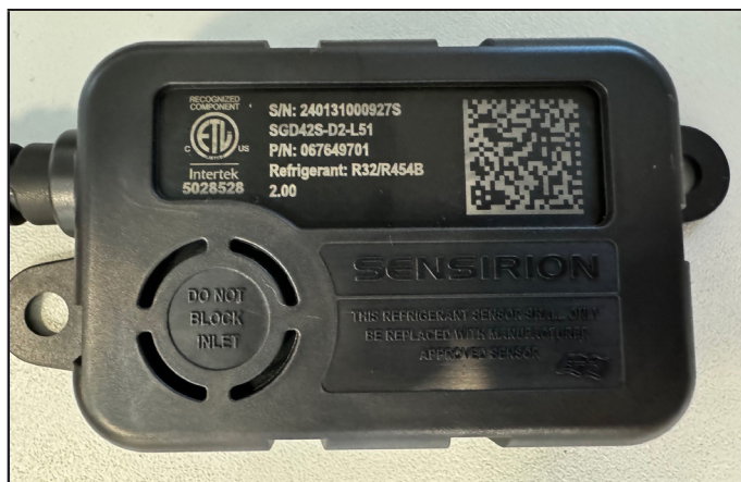
FIGURE 22. Example of Clear, Unobstructed Sensor Inlet
