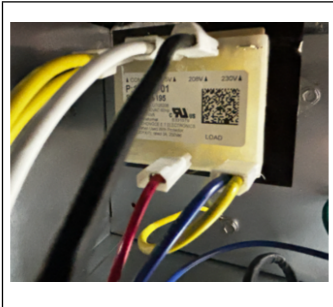
Figure 25. 230 TO 208 Voltage Conversion
