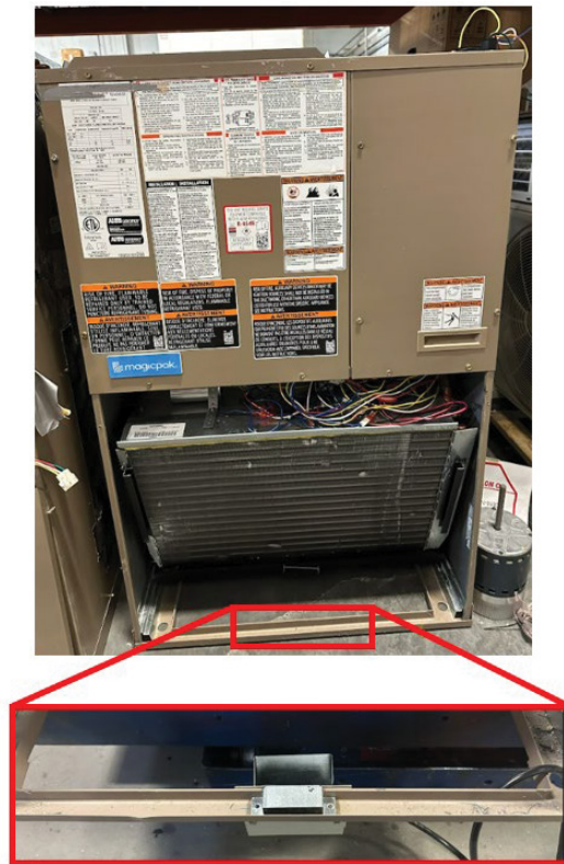
RDS Sensor Installation
