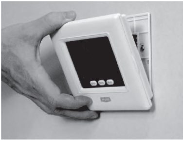
Fig. 4 - Attach Thermostat to Backplate
