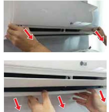
Figure 45: Removing the Bottom Cover, Alternate View.
