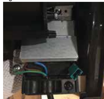
Figure 86: Terminal Cover Down.
