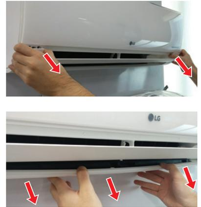
Figure 18: Bottom Cover with Top and Middle Unsnapped, Front View (Appearances May Vary Depending on Indoor Unit Model).
