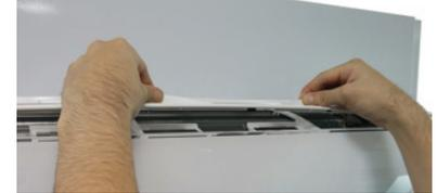
3. Disassembling the Air Filter.
