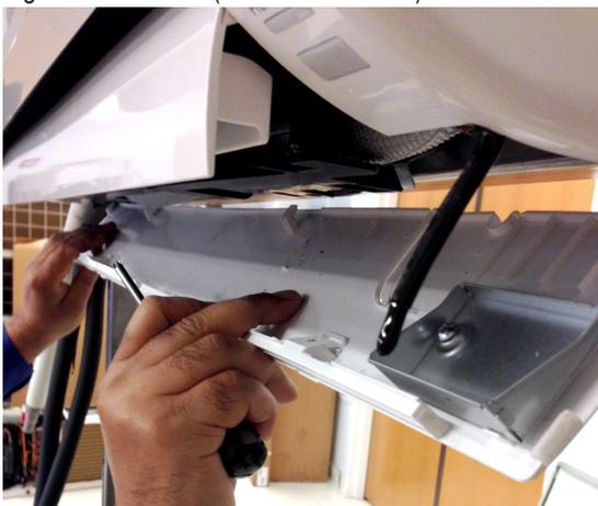
Figure 94: Latch over Screws on Bottom Panel, Indoor Unit
