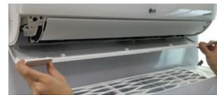
Figure 110: Securing the Bottom Cover C-hooks to the Indoor Unit Sockets (Step 3).
