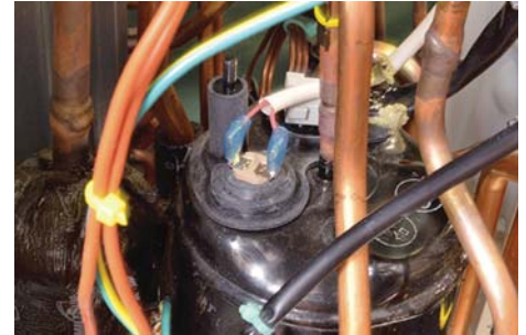
Compressor Overload
