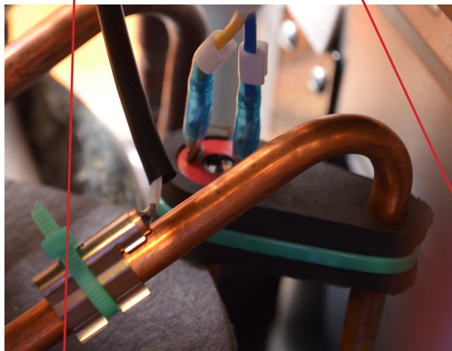
Discharge Temperature Sensor
