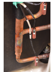
Gas Valve Temp Sensors
