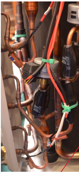
Liquid Valve Temperature Sensors
