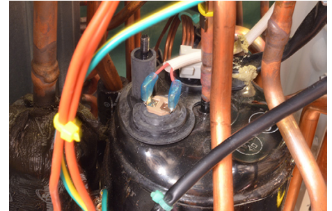
Compressor Overload
