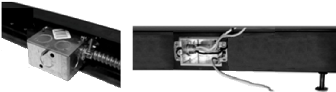
Figure 7 – Attach Conduit to Junction Box
